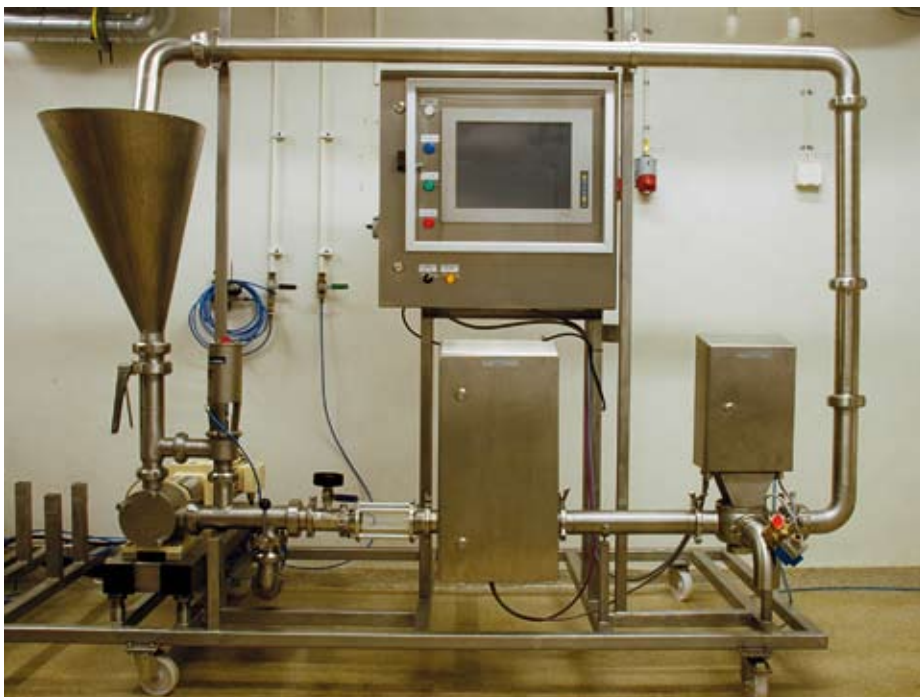
Picture 7: "Pilot plant at Food Radar Systems in Gothenburg, Sweden"
